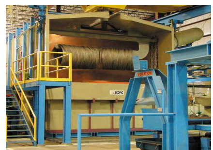
Acid Pickling for oxide removal.
