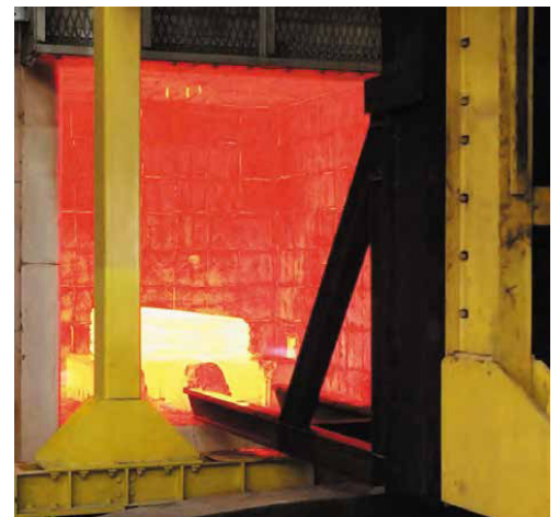
Batch annealing furnace
